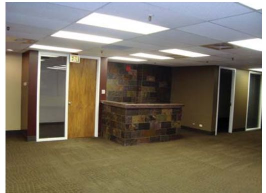
Built-in Reception Counter
