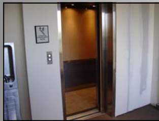
Lobby Upgrades Underway
