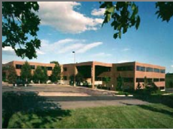
Building Exterior—Signage Available!
