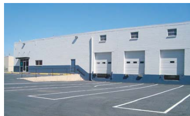
6201 EAST 42ND AVE Warehouse/Distribution
